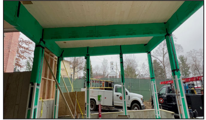
2. Wrap post/columns with WallShield IT to protect against moisture, mold, and construction damage. Use VaproTape to hold seams together when required, add corner protection (by others).
