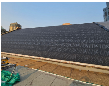
Standing Seam Metal Roof Optional use of VaproShim SA Self-Adhered under metal roof clips creates increased airflow under metal panels.
